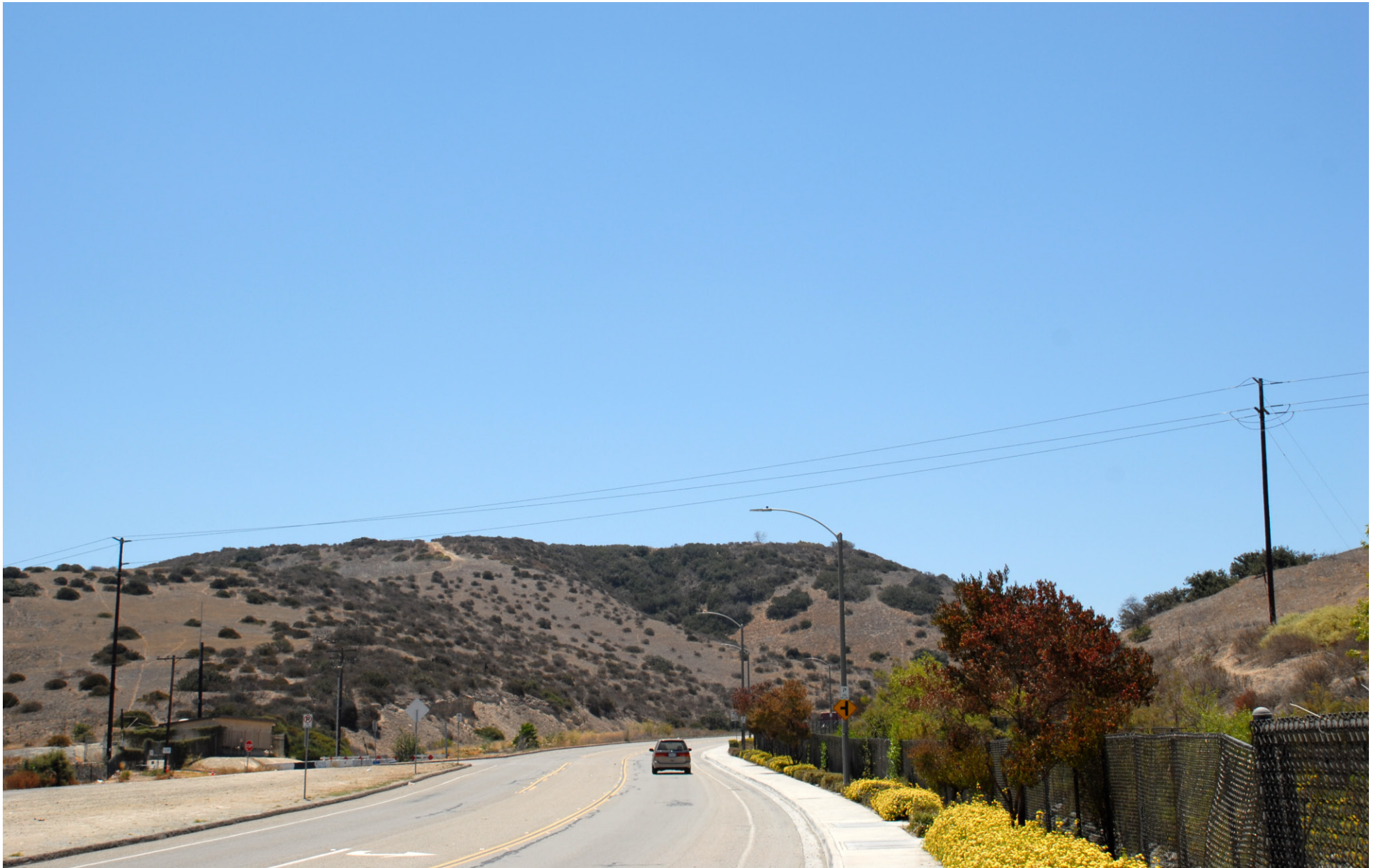
Existing view looking south from Heritage Road See Figure 4.1-1 for viewpoint location
