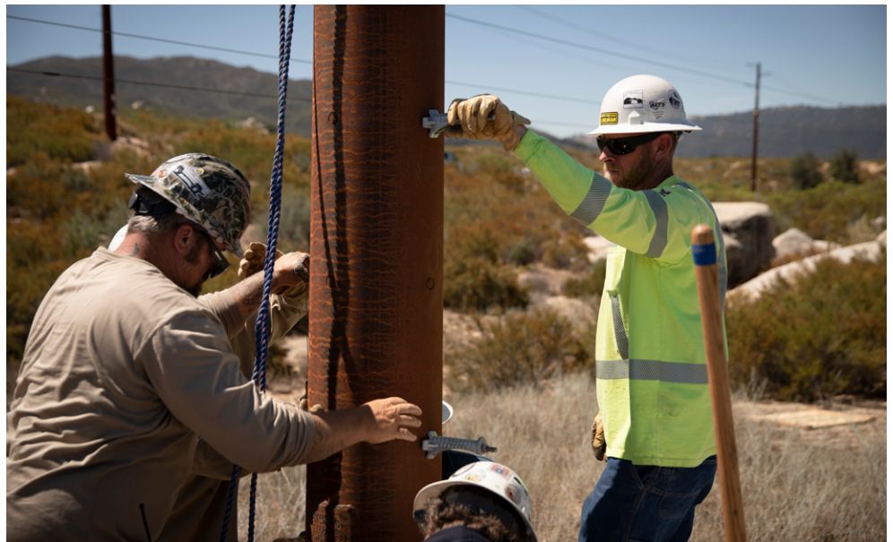
Wood-to-steel pole replacement project
