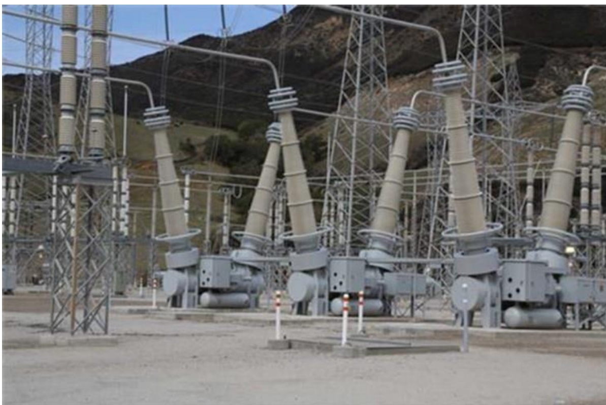
FIGURE 2-3 500 KV SWITCHYARD
