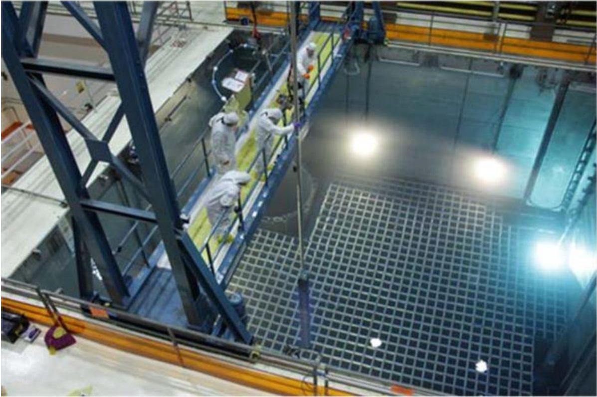
FIGURE 2-2 NUCLEAR FUEL OFFLOAD AT THE SPENT NUCLEAR FUEL POOL IN THE NUCLEAR FUEL HANDLING BUILDING
